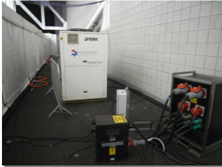
In the athletes tunnel- the 20kw AHU's can be seen
