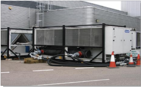
The completed installation
