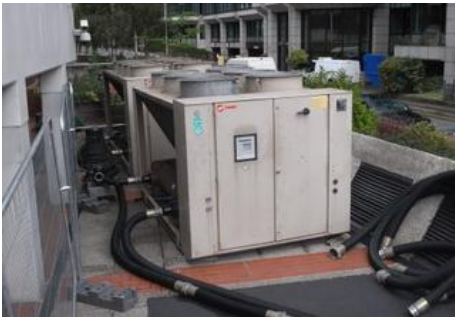
The completed installation
