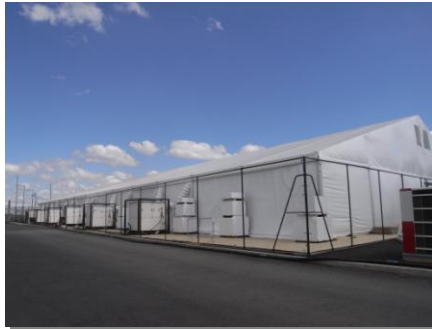
This was a big structure measuring over 70x 30mt in footprint
