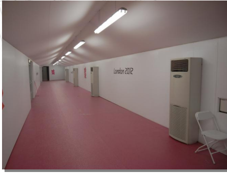
In the athletes tunnel- the 20kw AHU's can be seen
