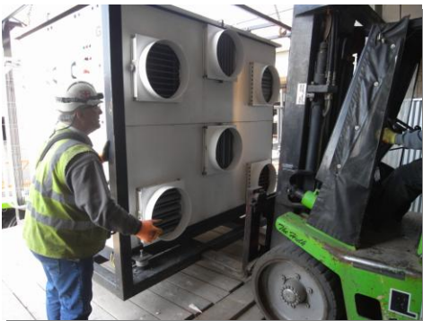
Offloading the truck on the ramp and positioning with a fork truck
