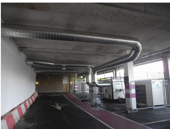
The completed installation- the air handler, spiral ducting and chiller can be seen
