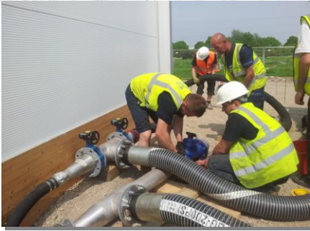
Installing the centralised water distribution system
