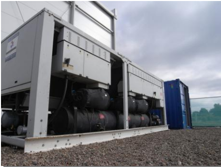
The completed chiller and pump station installation
