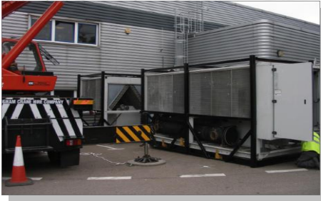
Chiller sections being installed
