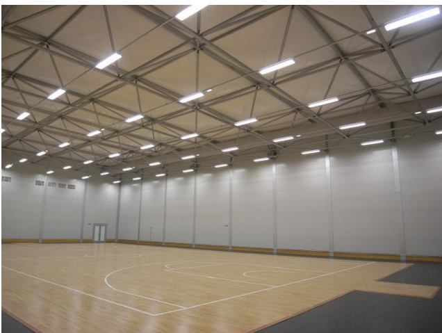
Internal shot of one of the completed basketball courts. One of the 800mm air socks can be seen to the rear
