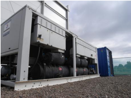
The completed chiller and pump station installation
