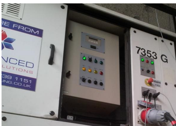
The controls section of an ACS Climate Control Unit
